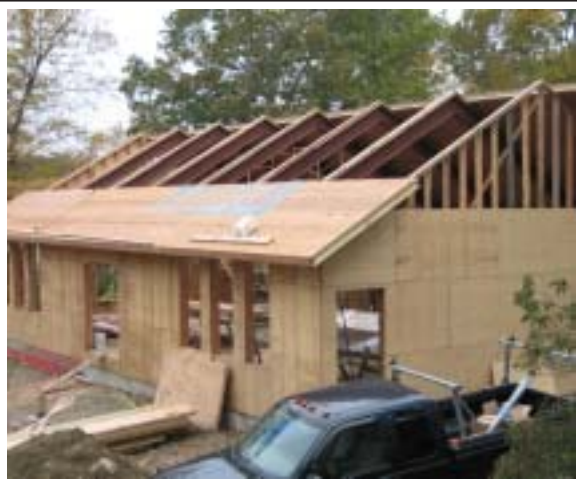
The new building is really started to take shape.
